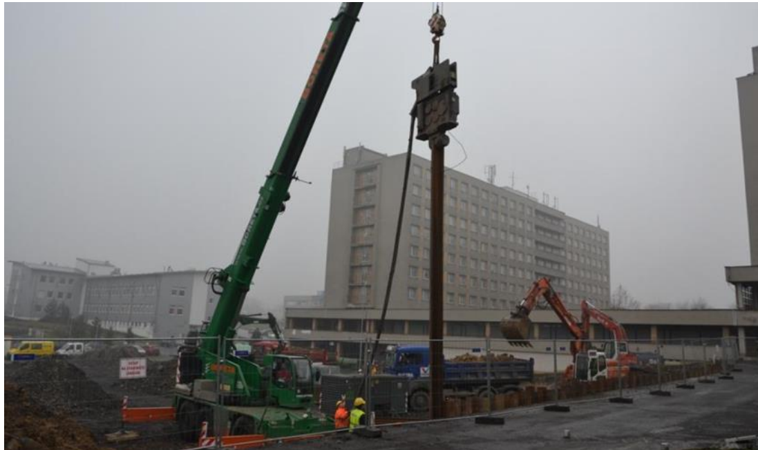
Fig. 6 Workplace preparation of foundation pit for supercomputer centre (photo: Stolárik)
