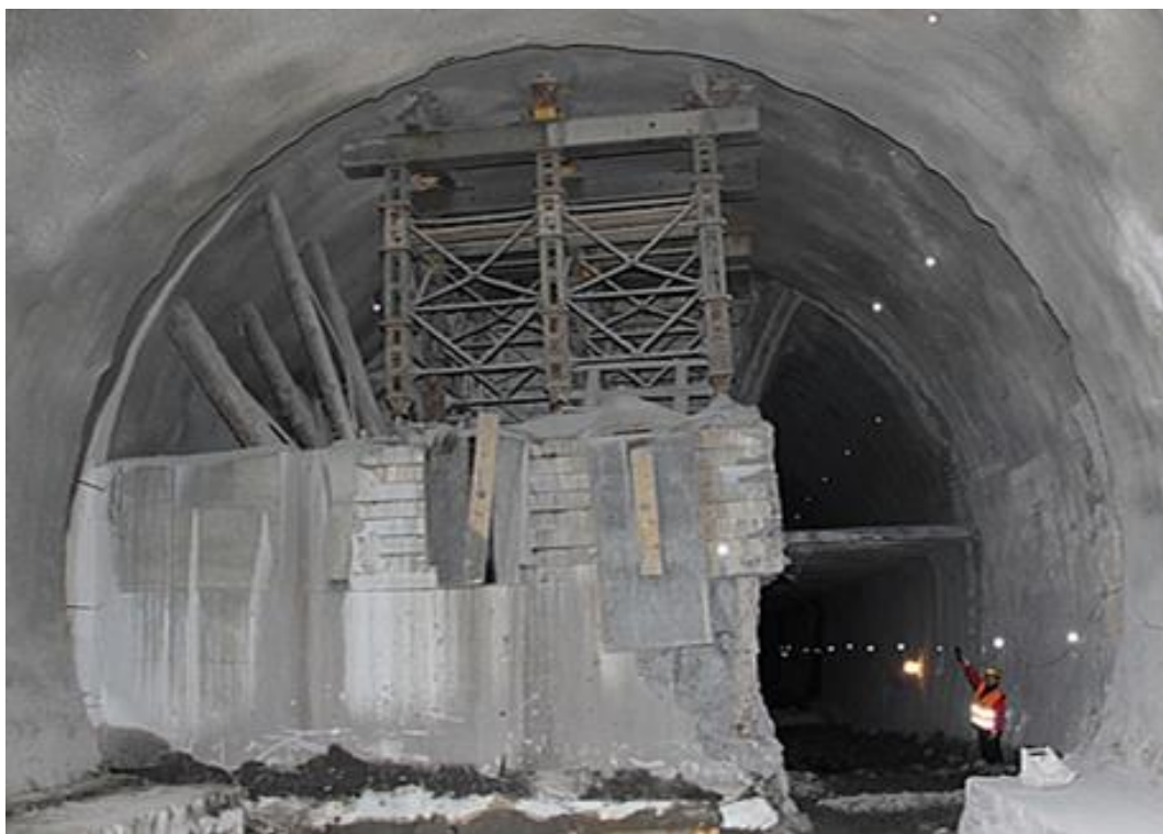
Fig. 2 Reconstruction of Jablunkov tunnel No. II (photo: Stolárik)
