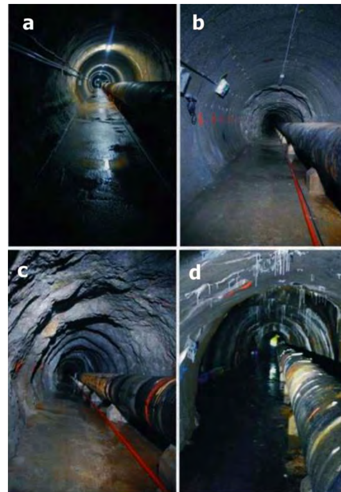
Fig.1 Different parts of the tunnel (explained in the text)
