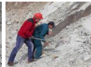
*Fig. 7b The borehole charge*
