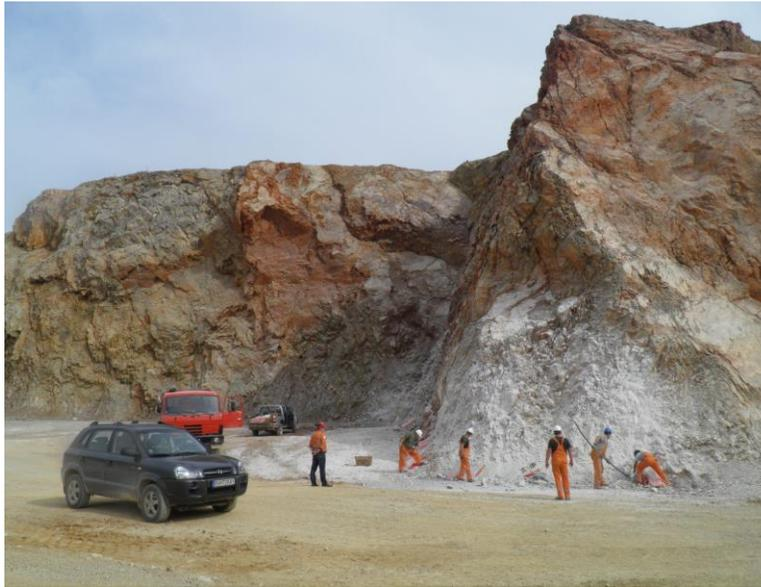
*Fig. 8a Charging and feeding of individual boreholes for the bench blasting No. 3873*
