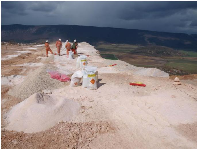
*Fig. 9a Charging and feeding of individual boreholes for the bench blasting No. 4049*
